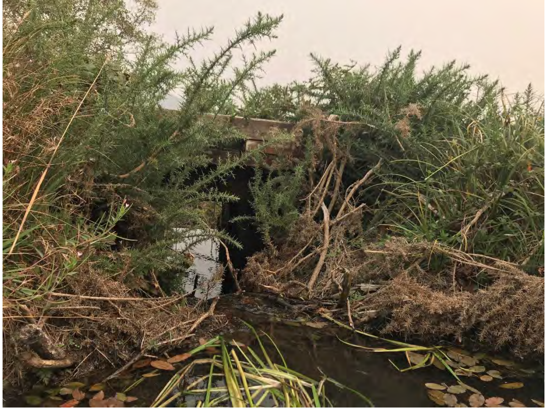
Photo 5: Former fire suppression pond culvert located at the north end of pond, facing north, draining into Bagley Creek.
