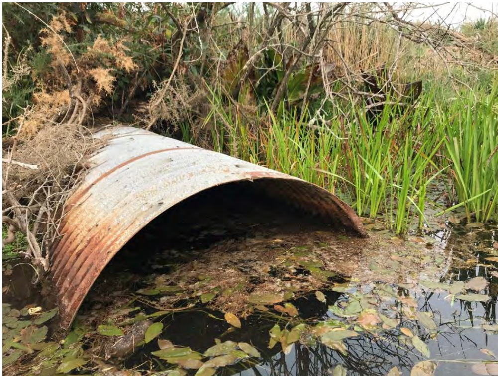
Photo 6: Culvert located at the south end of the former fire suppression pond, facing south.
