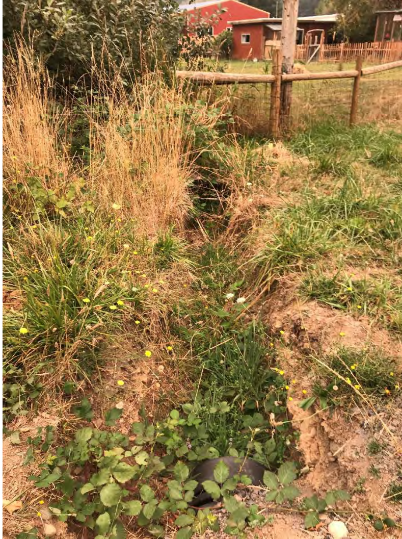
Photo 21: Culvert and swale, facing east.
